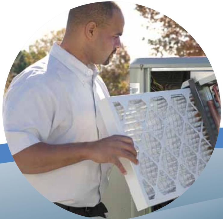
Proper filter maintenance is crucial to keeping HVAC ductwork clean. If dirt accumulates in the ductwork, and if the relative humidity reaches the dewpoint (so that condensation occurs), then bacteria and mold may grow. This is especially the case in HVAC systems with acoustical duct liners, which are frequently used in air handler fan housings and supply ducts to reduce sound transmission and provide thermal insulation.
