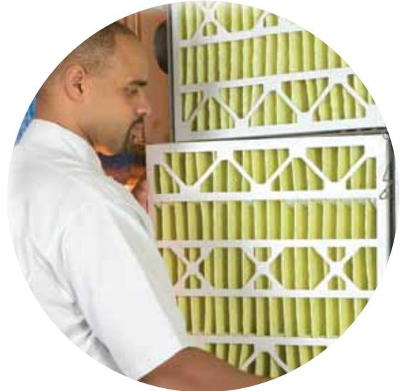
an open metal backing to support the media, panel filters today are made in much the same way they were made 75 years ago. Their simple construction and low filtration efficiency makes them among the lowest priced filters in use today.
